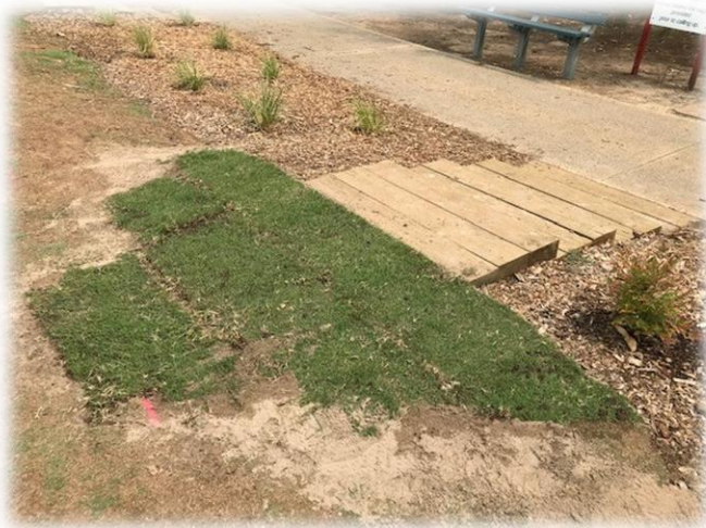
Turf work at 3 rd tee steps...
